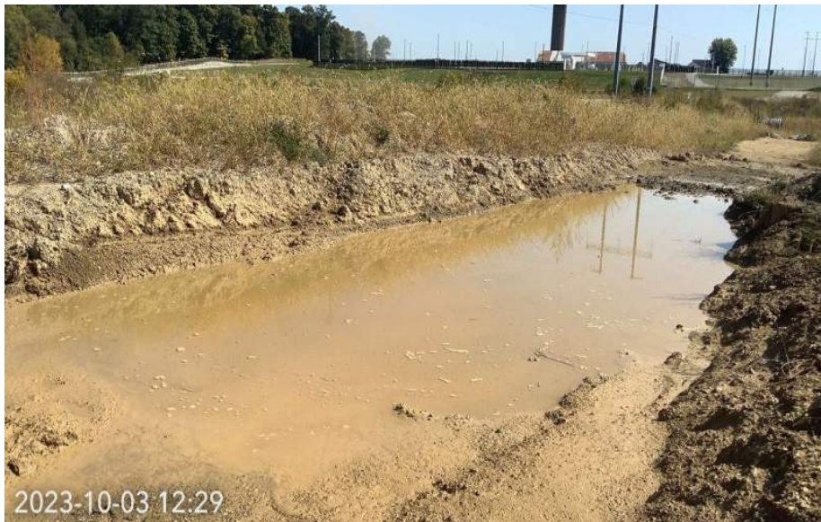
Photo Location 11. View of Open Water 4. Photograph taken facing southeast.
