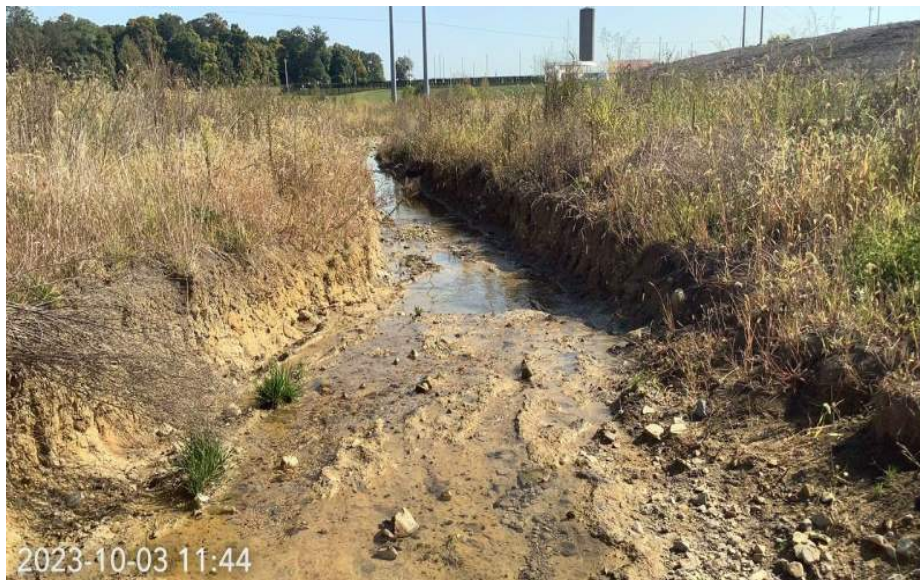
Photo Location 6. View of manmade upland drainage feature within the Project area. Photograph taken facing northeast.
